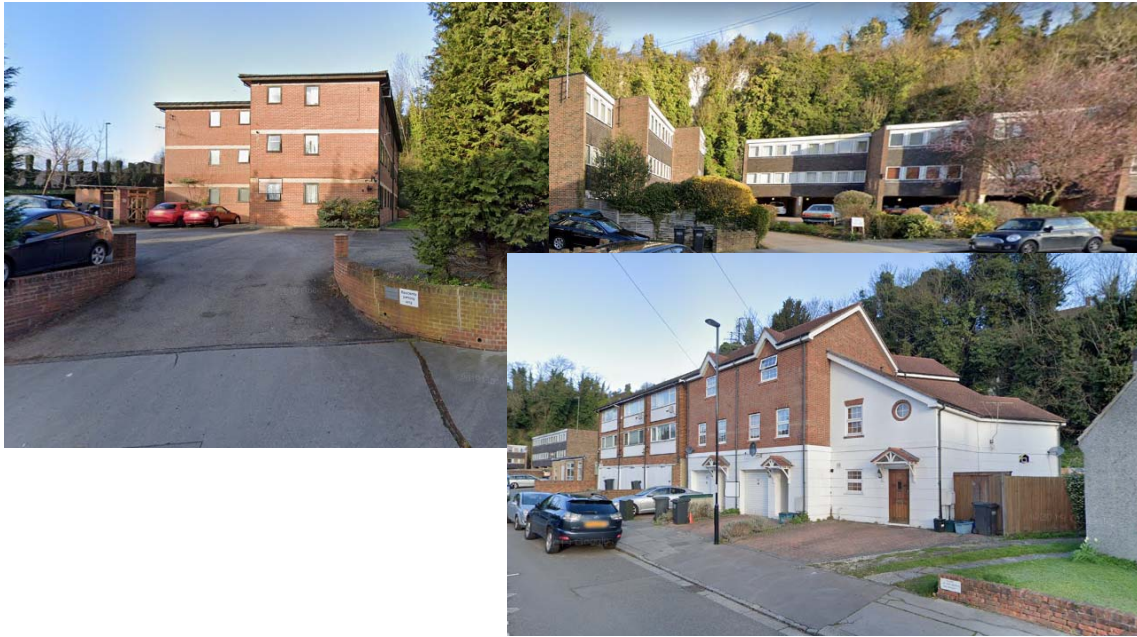
Figure 4 The surroundings areas character (137 – 165 Montpelier Road – top left, Dell House – top right and Cliff House/30/30a and 30b Biddulph Road – bottom right).
